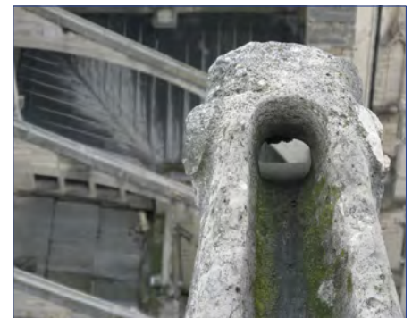
This gargoyle, overlooking some flying buttresses, was one of a plethora of medieval drain spouts jutting from the cathedral walls, designed to protect the walls from flowing water damage.
