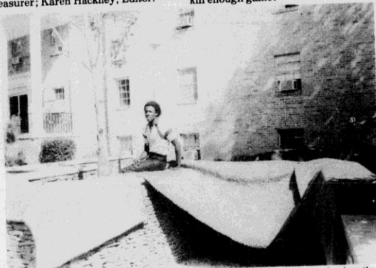
SURVEYING WATER-DAMAGED CARPETS—Shawn Williams checks the progress of drying carpets which were soaked by up to four inches of water seepage in the Haskel Lucas basement.
