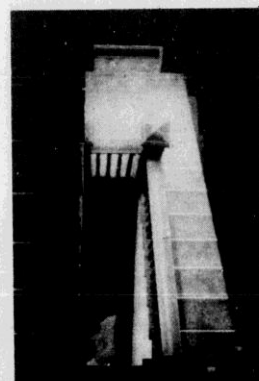
SOLID PINE was stained then used to construct this stairway which goes up three floors and down to the basement. Except for dust, most of the stairs are as fit to walk on today as they were years ago.
