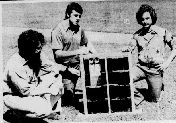
DR. WILLIAM (Bill Hayes, Donald Clift and Mark Youngker reveal the aluminum can composition of PTK's prize-winning solar radiation collector.
