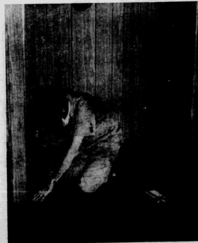
INSTRUCTOR VERNON HURST lays down carpet to add to the finishing touches of the Faculty Lounge located in the basement of Fulton Hall. All work on the lounge was provided by volunteers, and as soon as the lounge is finished, they will begin work on the Commuter Lounge.
