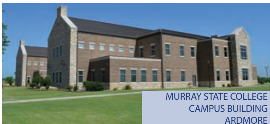
MURRAY STATE COLLEGE CAMPUS BUILDING ARDMORE
